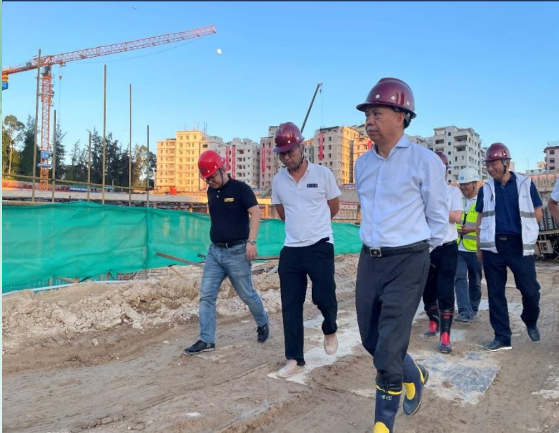
Daytime construction inspection
