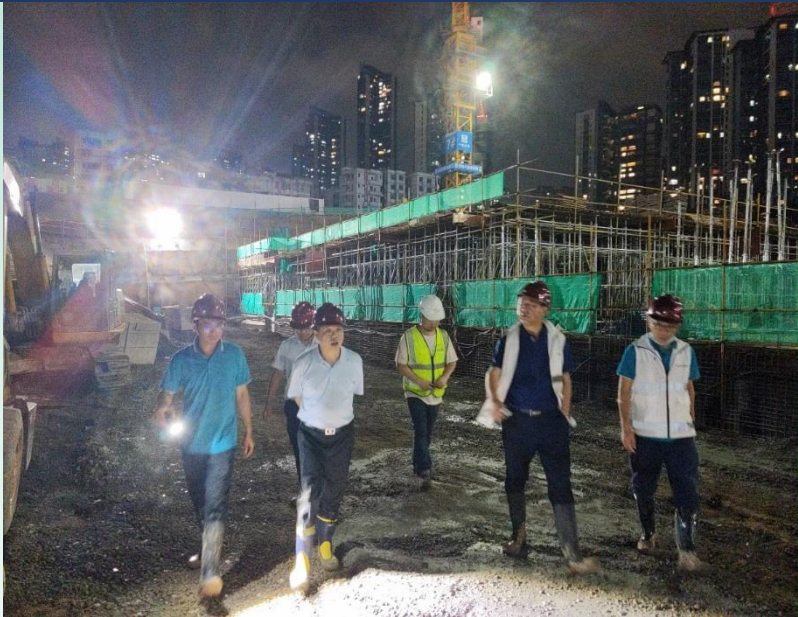
Night construction inspection
